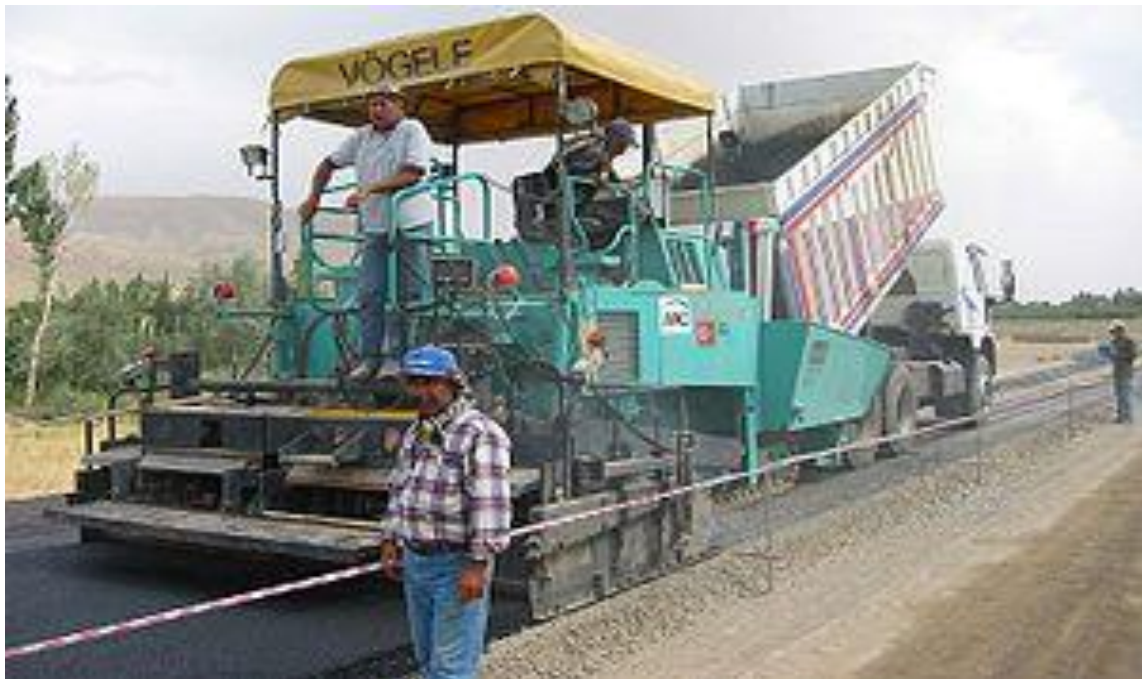
Fig.2 . A machine laying asphalt concrete, fed from a dump truck
