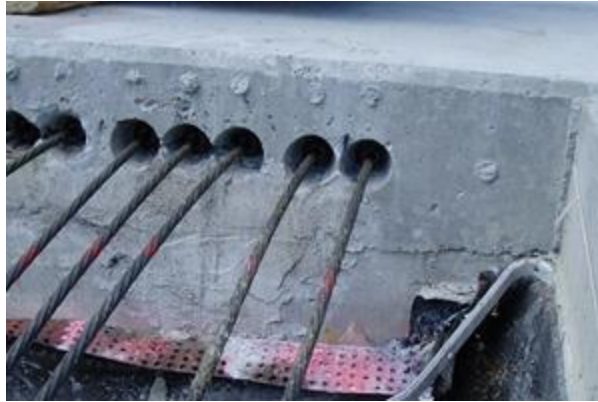
Tendon (cable) tails after tensioning
