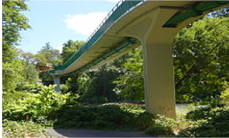
Stressed ribbon pedestrian bridge, Grants, Oregon, USA
