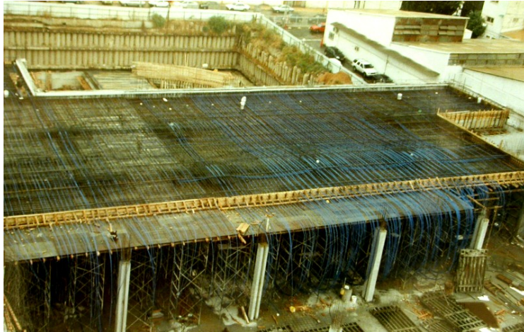
Part of the slab before placing the concrete
