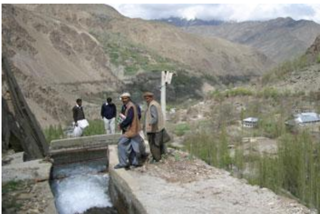
(Fig.4) (Micro-hydropower projects permit significant villager involvement in all phases of the work).
