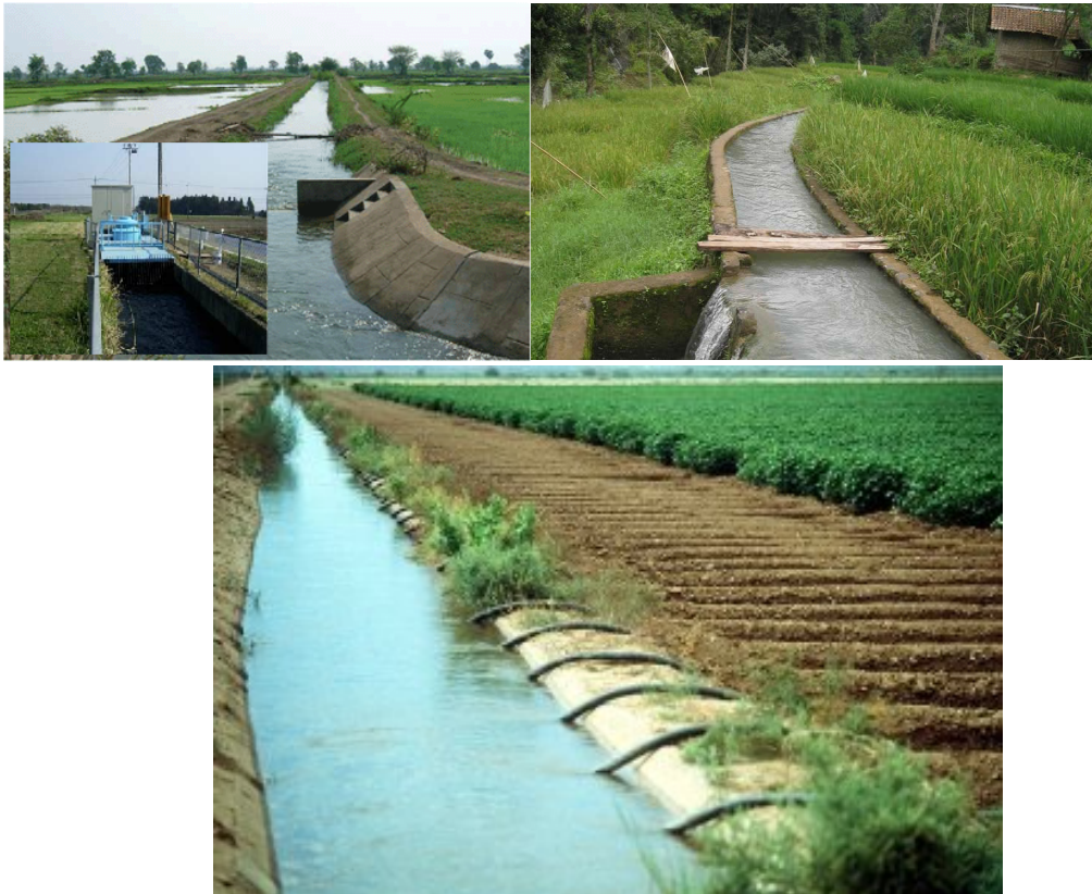
(Fig.3) (This micro-hydropower plant is integrated with an irrigation scheme, using excess water to generate power for a nearby town, thereby displacing the diesel fuel that would otherwise be used).
