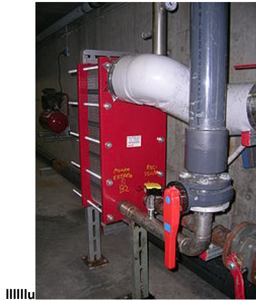
An interchangeable plate heat exchanger applied to the system of a swimming pool
