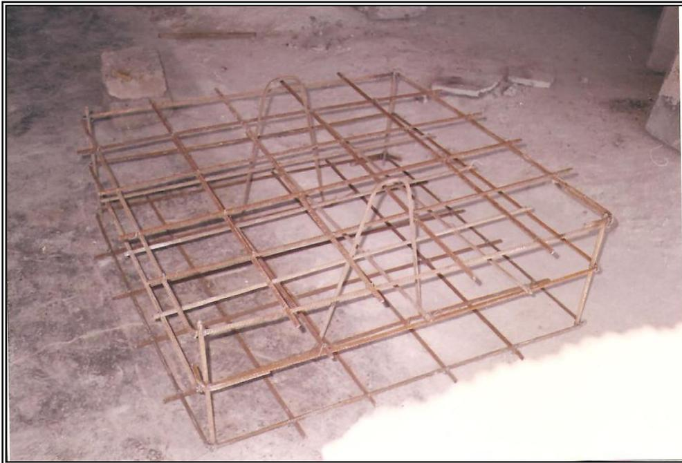
*Plate (4.1) Reinforcement of the Footing*
