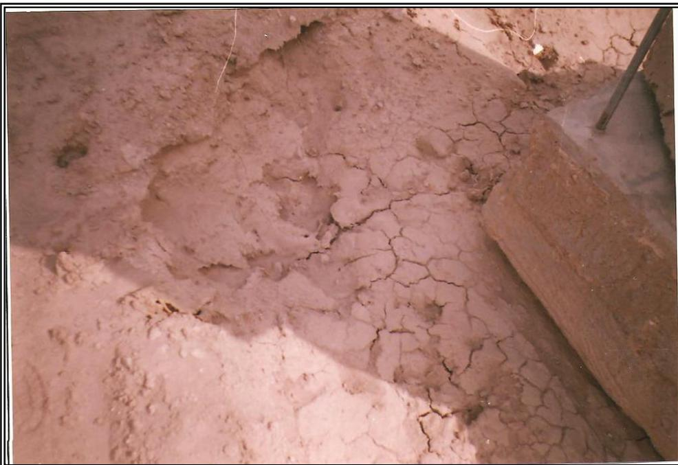
*Plate (5.2) Sinkholes around the Footing*
