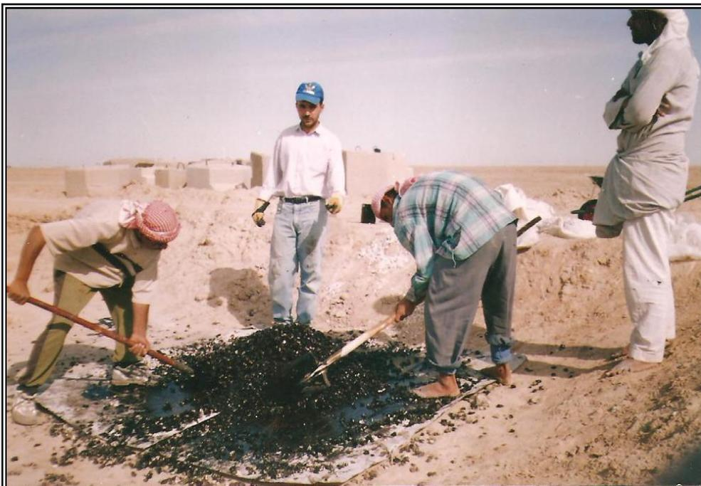
*Plate (4.5) Material Mixing Stage*
