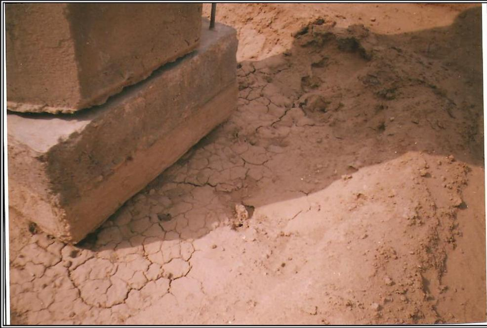
*Plate (5.1) Sinkholes around the Footing*
