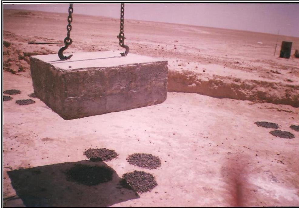
*Plate (4.7) A Typical Footing during Handling and Place in Position*
