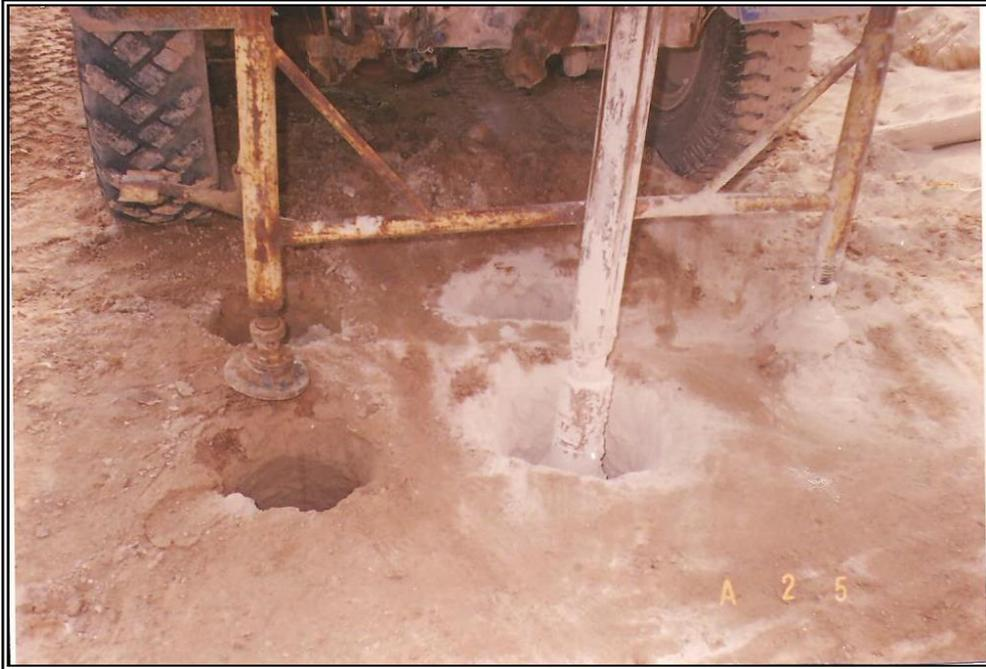
*Plate (4.4) The Four Holes after the Completion of Drilling Process*
