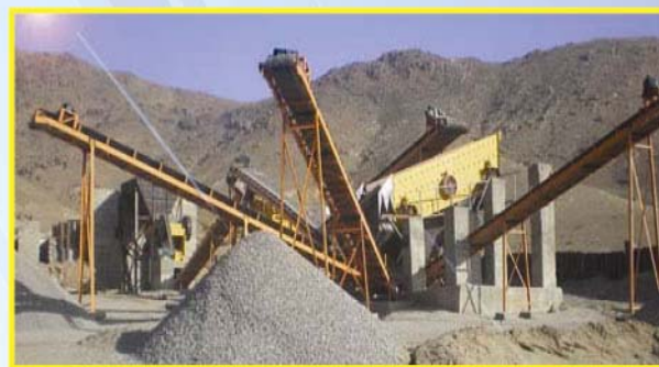
Figure 2 : Aggregate Production Equipment (Stone Crusher)
