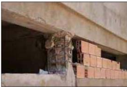
Figure 19. Captive column damage from (a) 2003 Bourmerdes, Algeria earthquake (photo: M. Farsi), and (b) 2001 Bhuj earthquake in India. (source: EERI)
