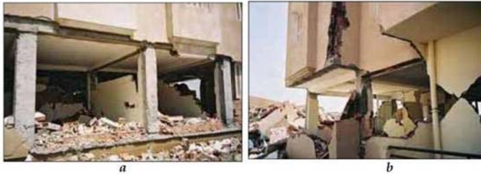
Figure 15. RC frame building with masonry infills in Algeria (after the 2003 Boumerdes earthquake): (a) masonry infill walls fail in both directions; (b) Masonry infill wall failure showing diagonal cracking due to compression strut action (photos: S. Brzev)
