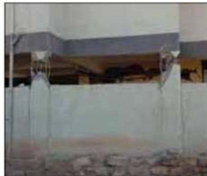
Figure 19. Captive column damage from (a) 2003 Bourmerdes, Algeria earthquake (photo: M. Farsi), and (b) 2001 Bhuj earthquake in India. (source: EERI)
