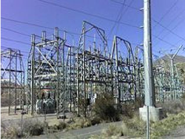
A transmission substation decreases the voltage of incoming electricity, allowing it to connect from long distance high voltage transmission, to local lower voltage distribution. It also reroutes power to other transmission lines that serve local markets. A transmission substation may include phase-shifting or voltage regulating transformers. This is the PacifiCorp Hale Substation, Orem, Utah, USA.
