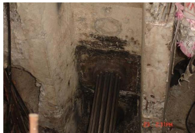
FIGURE (۳) CASTING CONCRETE WITH GLASS FIBRE SURROUNDS PRESTRESS STRAND CABLE AT HOLAKAR BRIDGE
